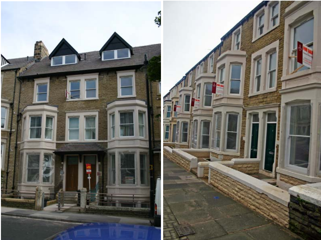
Fflat conversions on West End Road and remodelled family homes on Clarendon Road East
